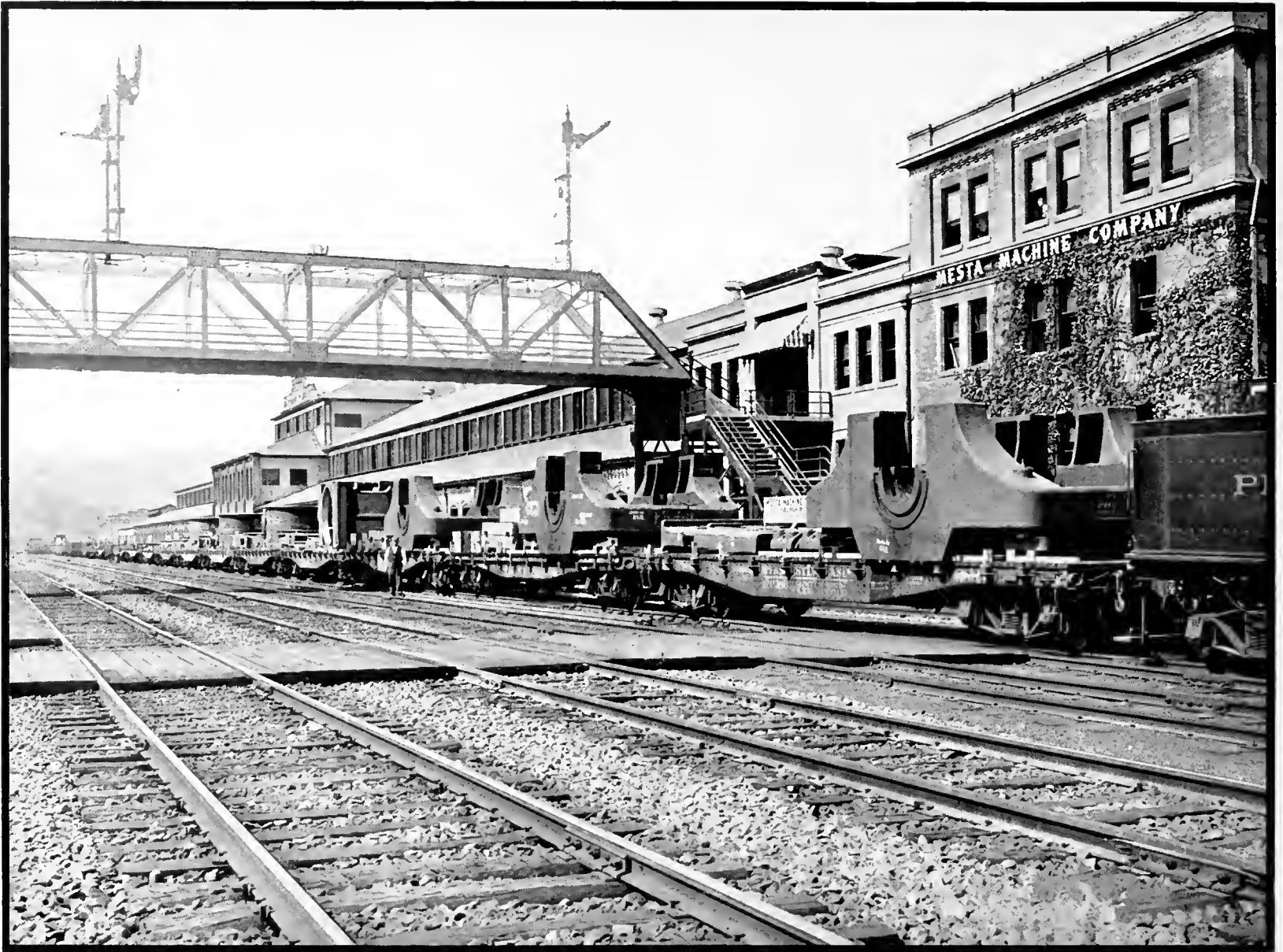
Shipment of Three Vertical Long Crosshead Type Blowing Engines for Export
